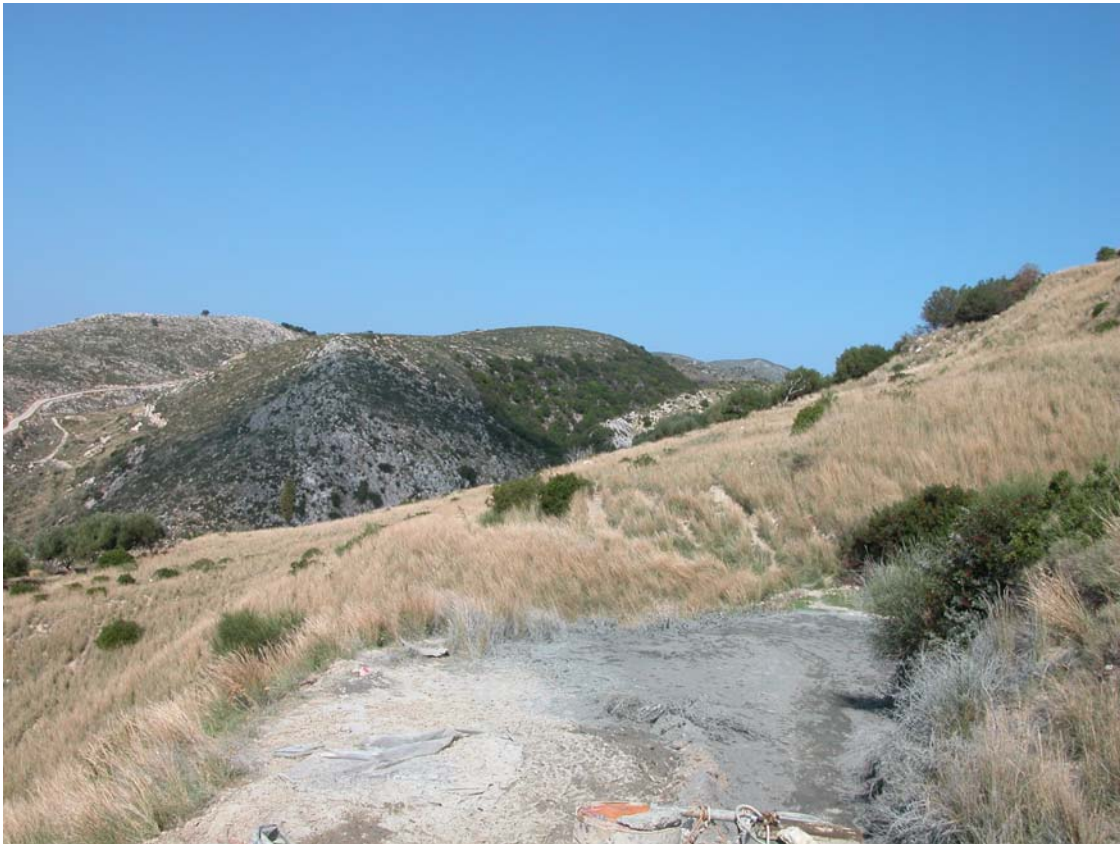
Figure 8: Road interrupted by landslide and slumping A connecting road is also interrupted on the other side of this landslide
